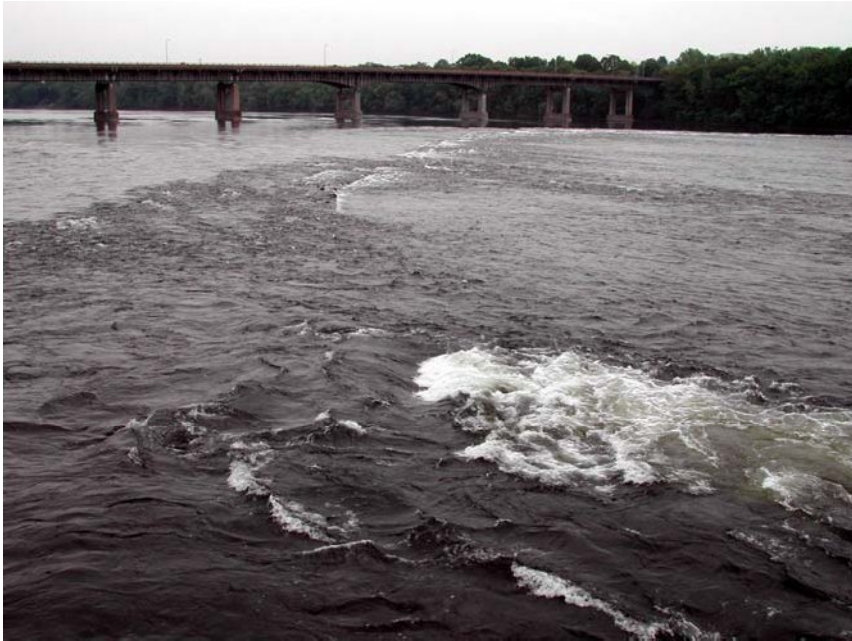
Enfield Dam from the western shore, looking upstream. River flow at the time the photograph was taken was approximately 14,000 cfs.
