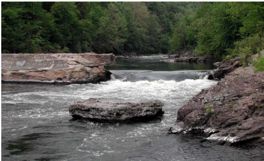
Lower Tariffville Gorge, looking upstream through breached concrete dam. Flow at the time the photograph was taken was approximately 700 cfs. Vertical drop through the dam was approximately 1.75 m, with an estimated maximum velocity of 2.5 \text{ m} \cdot \text{sec}^{-1}
